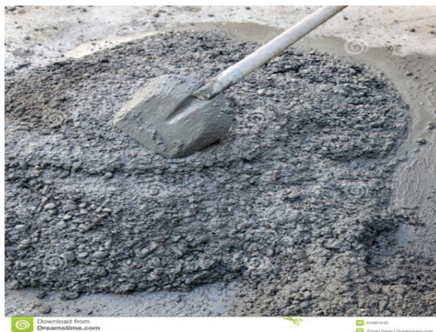
Figure 3. Mixing Of Concrete
