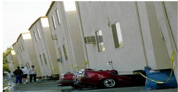
**Figure 1** Soft storey failure
