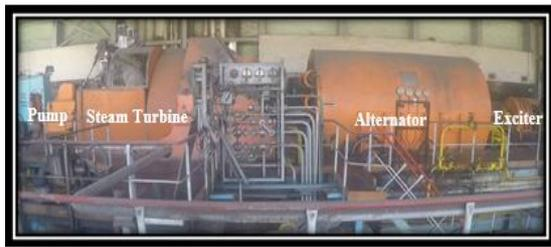
**Figure 1** Picture of the turbo-alternator group
